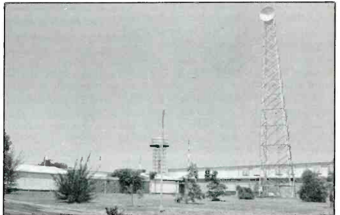
The RA transmitter site at Darwin.
